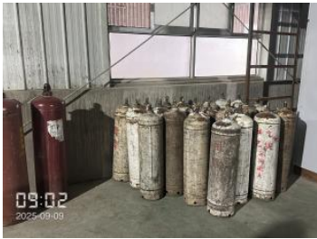
cylinders were not fixed and without cylinder caps.JPG
